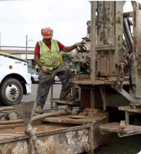
Drilling vertical wells for geothermal instructional system
